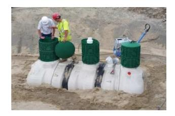
☐ Step 8: Locating and Installing Air Pump/Control Panel.
