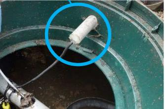
☐ Step 11: The FujiClean Treatment System must be vented. In most cases, the system will vent through the building's septic discharge pipe and building plumbing. In cases where there is a blocked air way (e.g. effluent pump), or in severe downdraft locations, a separate vent should be installed. If you install a vent, be sure that the vent pipe slopes toward the tank so that any moisture accumulation drips toward the tank.
