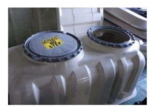
Use sharp blade to remove inner plastic ring.
