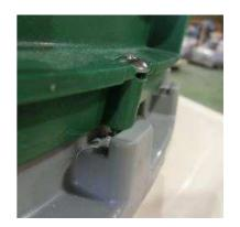
Tuf-Tite Risers. Align riser screw holes with molded "frame block" and screw tight. Maximum screw length is 1 ½"
