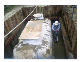
□ Step 6 continued: Install inlet and outlet pipes using primer and cement. For larger systems with 5" inlet and outlets, you may use 5": 4" eccentric reducer adapters included with system. (Except CE14) Install with thin edge down. Apply primer and cement to 4" PVC pipe sections to inlet and outlet.
