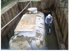
□ Step 6 continued: Install inlet and outlet pipes using primer and cement. For commercial systems with 5" inlet and outlets, you may use 5": 4" eccentric reducer adapters included with system. (Note: CE14 units have 4" inlets and outlets). Install adapters with thin edge down. Apply primer and cement to 4" PVC pipe sections to inlet and outlet.
