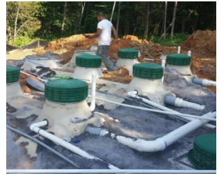
Systems may be clustered in parallel configuration for treatment of larger flows.
