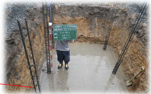
Rebar with Adhesive
